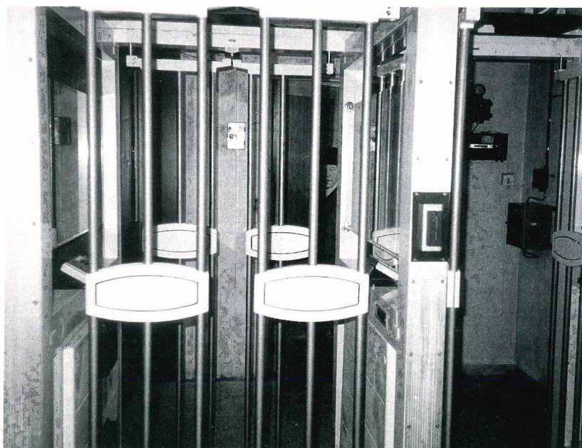
"MANTRAP" produced in Russia and installed at the Kurchatov Institute of Atomic Energy, Moscow, with funding from the US DOE's lab-to-lab cooperative program on fissile materials security. To open the outer gate a person must insert a magnetically coded ID card into the reader on the right. Before the individual can pass the inner gate, the personal ID number typed into the keypad on the left inner wall and the weight determined by a scale in the floor must agree with the ID card. As the person exits, sensors detect any low-energy gamma radiation from highly enriched uranium or any metal that might shield these gamma rays. Anyone not passing these tests is locked between the gates. (Courtesy of Sandia National Laboratory.) FIGURE 3
