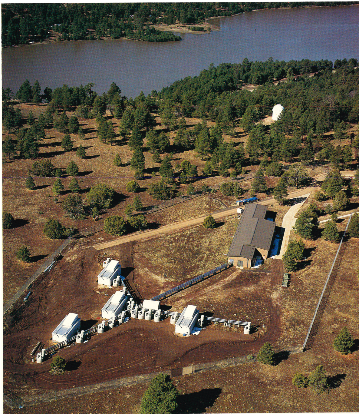
NAVY PROTOTYPE OPTICAL INTERFEROMETER at Lowell Observatory on Anderson Mesa, Arizona. The small white buildings seen in this aerial view house the elements of the astrometric array; the six imaging array elements will be moved among the concrete piers along the arms of the Y. The long building is the optics laboratory, housing the delay lines. Also visible are one of the Lowell Observatory domes and Lower Lake Mary, about 200 feet lower than the top of the mesa. FIGURE 1
