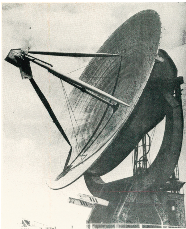
Ruby maser mounted in 1957 at the focus of the 50-foot radio antenna on the roof of the Naval Research Lab in Washington, DC. Built by Lee Alsop, Joseph Giordmaine and Townes at Columbia, this was the first maser to be used as an amplifier for radioastronomy. Figure 2
