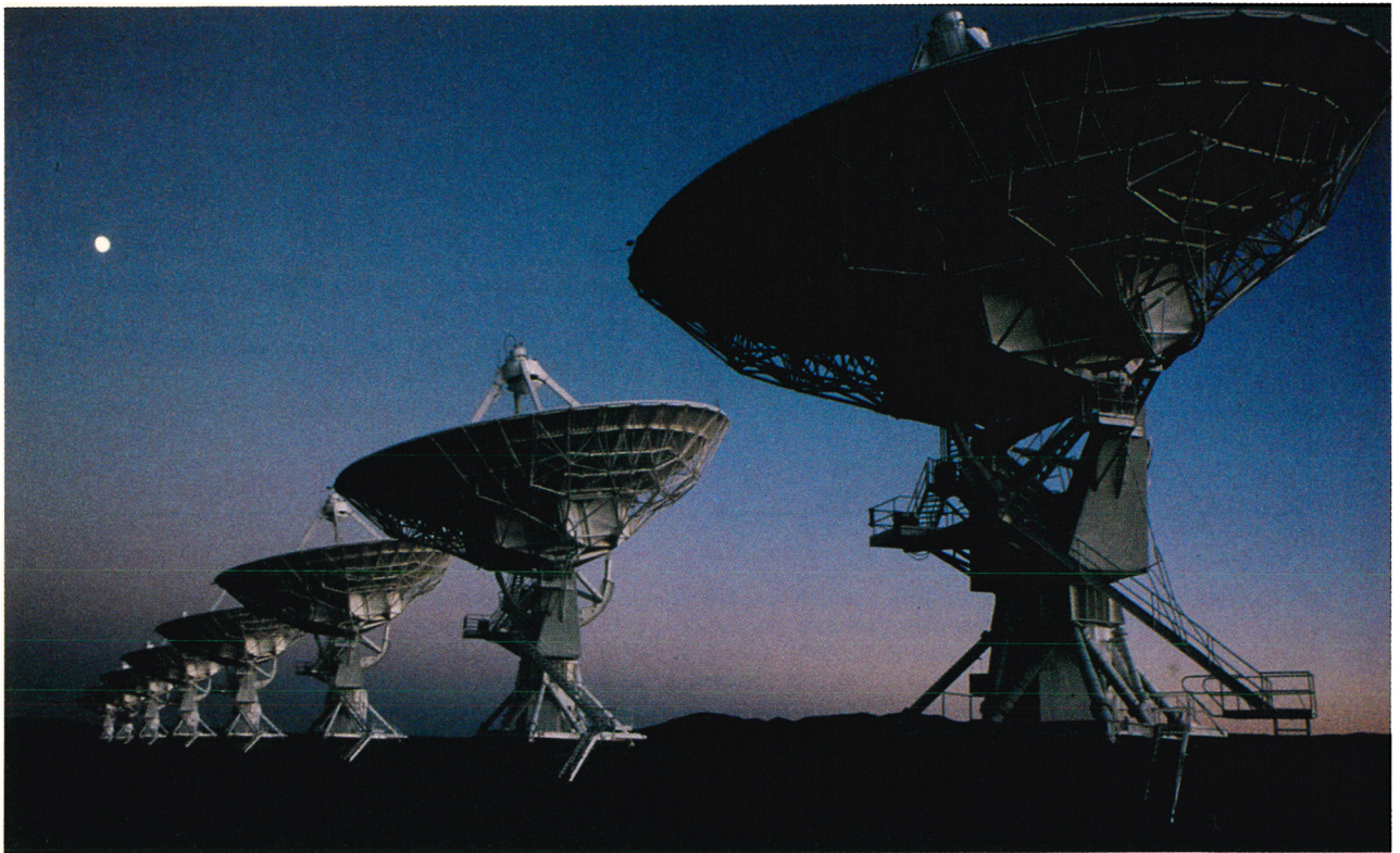
The Very Large Array of radiotelescopes in Socorro, New Mexico, is a Y-shaped string of 27 movable antennas that can range over 63 km of track. Interferometric techniques with such multiple-antenna systems can reduce sensitivity to radio interference by 20 dB. The VLA recently detected 3 the 1420-MHz atomic-hydrogen line enormously redshifted to 323 MHz. Figure 2
