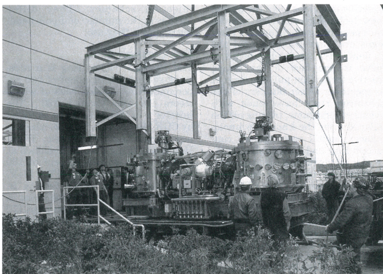
Helios compact synchrotron being guided into IBM's Advanced Lithography Facility after being shipped from the supplier, Oxford Instruments in England. This superconducting storage ring features two 180° bending magnets, seen at either end, that steer the electrons in a racetrack-shaped trajectory. The company is exploring the machine's potential as a commercial source of x rays for lithography.
