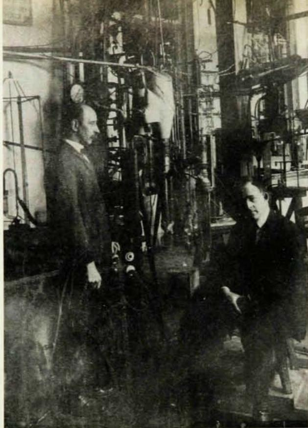
Cryostat for liquid helium containing the calorimeter that Dana used at Leiden. The cryostat is surrounded by concentric Dewar flasks that held liquid hydrogen and liquid air for thermal isolation. Figure 3
