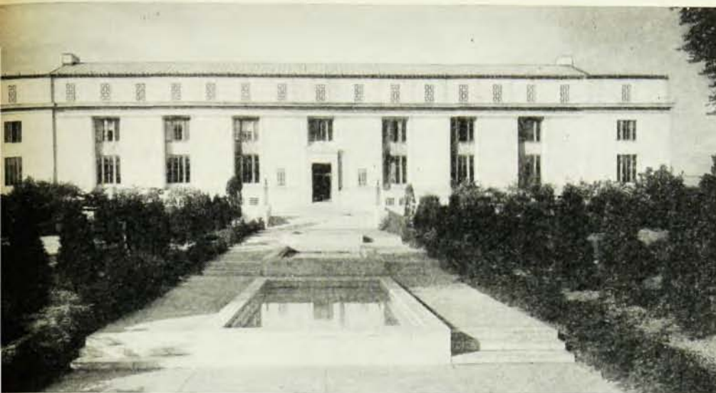
The National Academy of Sciences' building at 2101 Constitution Avenue, Washington, D. C., serves as the headquarters for the National Research Council.
