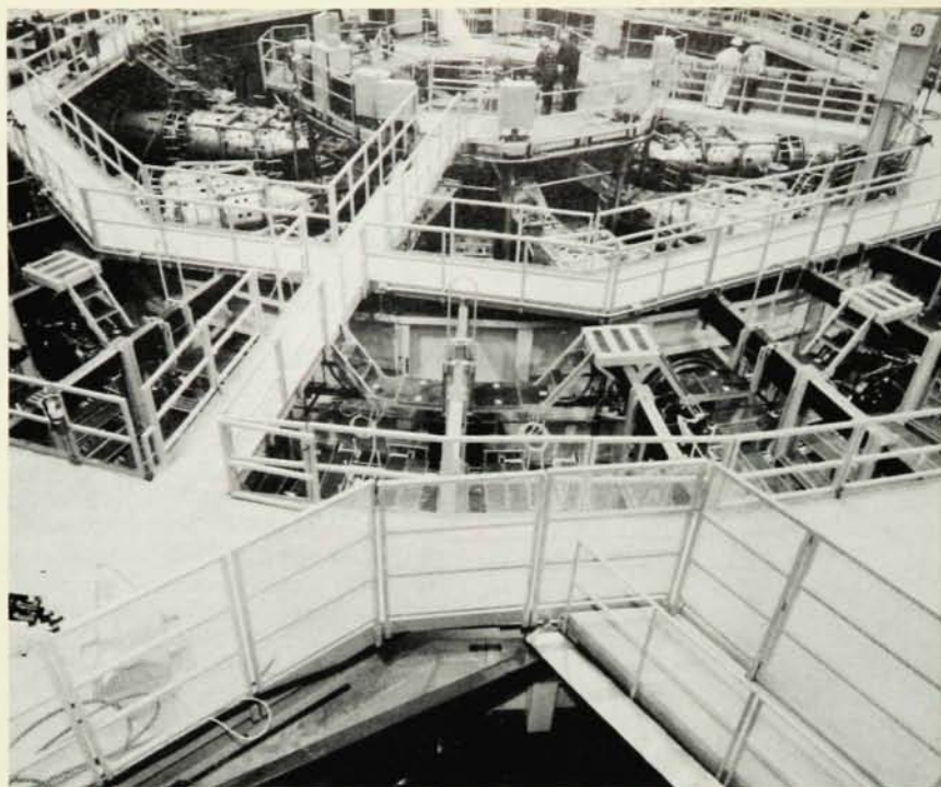
The light-ion-beam fusion accelerator facility PBFA-II, which began operation last December at Sandia, is the only existing inertial-confinement driver with sufficient energy to implode a D-T pellet to ignition—if major hurdles of pulse shaping and focusing can be overcome. Thirty-six pulse-power modules, radiating inward from a surrounding array of capacitor banks, will deliver 10-nanosecond voltage pulses to a small central diode, enabling it to accelerate 2-megajoule converging disk-shaped beam bursts of lithium ions toward the implosion pellet at its center.
