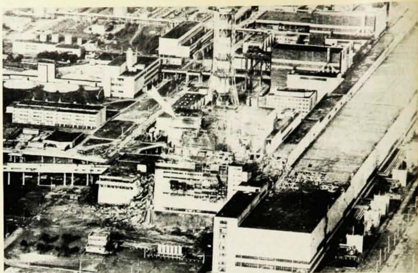
Chernobyl nuclear power plant a few days after the accident. The arrow indicates the damaged unit. (Photo from Tass, courtesy Sovfoto.)
