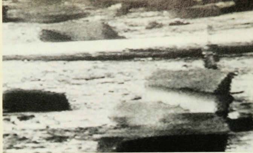
Debris thrown up by force of the Chernobyl explosion litters roof of adjacent building. A large chunk at right, in front of a length of 6" pipe, appears to be half of a graphite block, with indentation left by cylindrical cooling channel. (Photo from Soviet tv, provided by Ed Purvis.)
