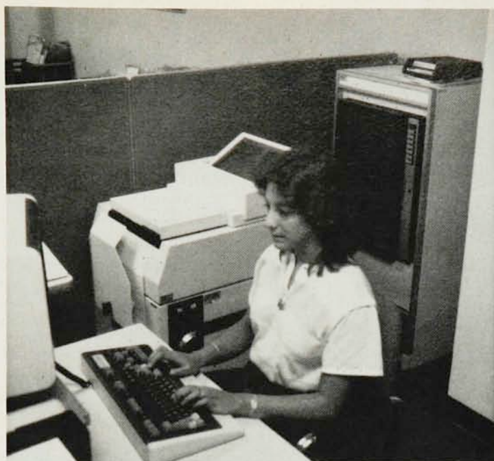
Kurzweil page scanner. This page reader converts typed manuscripts directly into Atex files, eliminating one stage of keyboarding. Because it "learns" how the typed characters of each manuscript should be interpreted, the Kurzweil scanner can read an extremely wide variety of typefaces.
