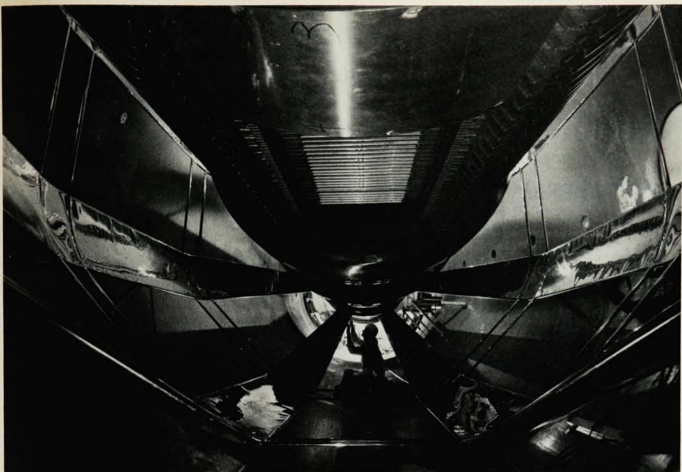
The Tandem Van de Graaff accelerator at Brookhaven is being upgraded in support of the Laboratory's relativistic-heavy-ion project for the Alternating Gradient Synchrotron. Looking along the high-voltage support column inside the Van de Graaff's (horizontal) pressure vessel, one sees the "portico intershield" being installed—eight radial panel structures that will provide higher voltage in normal operation and increased reliability at the 15-megavolt level necessary for injection of ions into the AGS. A tunnel to transfer ions from the Van de Graaff to the AGS is now under construction. The system would eventually serve as the source and injector for the ultrarelativistic heavy-ion collider Brookhaven proposes to build in the vacant CBA tunnel. Figure 7
