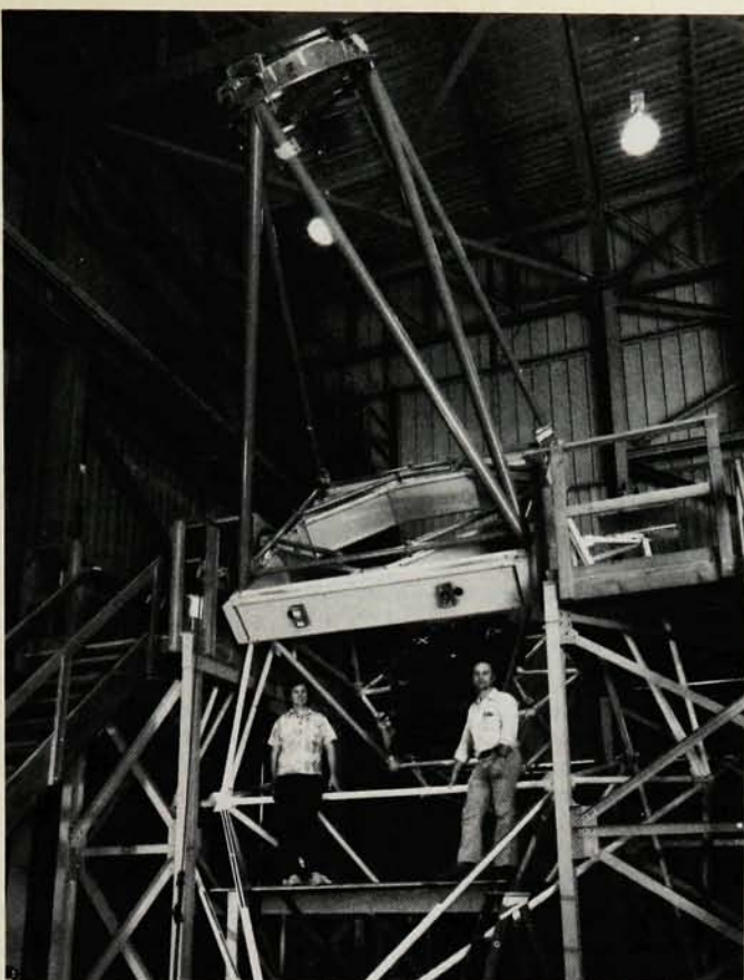
Demonstration instrument built at Lawrence Berkeley Laboratory to test the actuator and sensor systems for a segmented-mirror telescope. At the left of the mirror segment is Jerry Nelson, leader of the team that built the Technical Demonstration Telescope, and at the right is his co-worker George Gabor.
