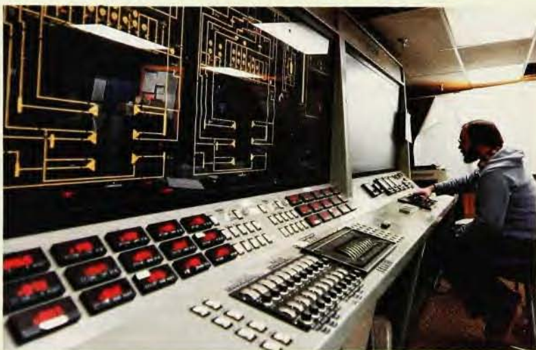
Helium flow (represented by yellow diagram) is monitored at the control panel of the Fermilab central helium liquefier facility. The central facility plus 24 satellite refrigerators provide 24 kW of cooling for the Tevatron's niobium-titanium superconducting magnets.
