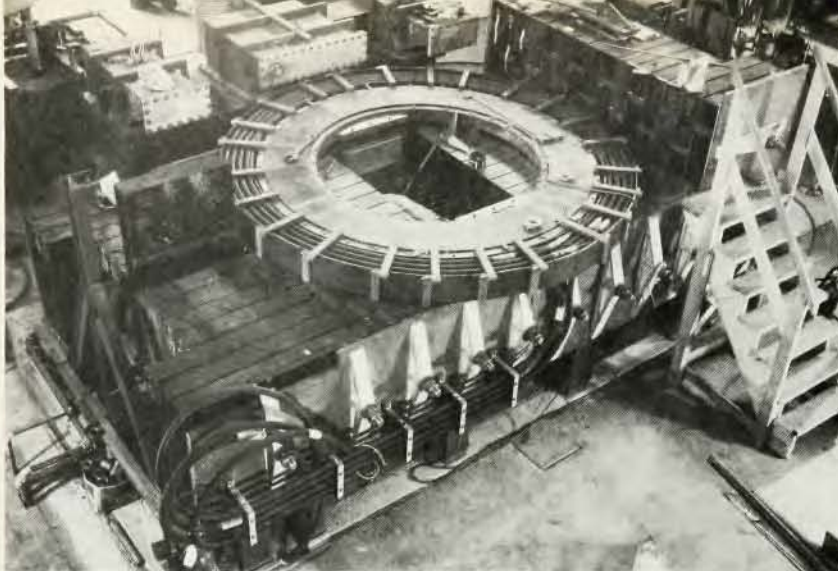
Lower yoke of the Berkeley synchrotron magnet and the coils that carry pulses of current from the condenser bank to excite the rectangular-design magnet. Figure 2
