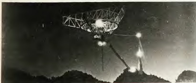
The radio telescope at Arecibo, Puerto Rico is sometimes used for SETI research. This figure shows the receiving antenna poised high above the 1000-ft.-diameter dish out of sight in the valley below. Photo courtesy of Cornell University.
