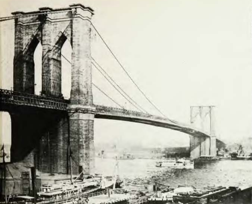
Brooklyn Bridge , pictured just before its opening in 1883, became a symbol of American ingenuity, heralding the new era of electricity with its many lights.
