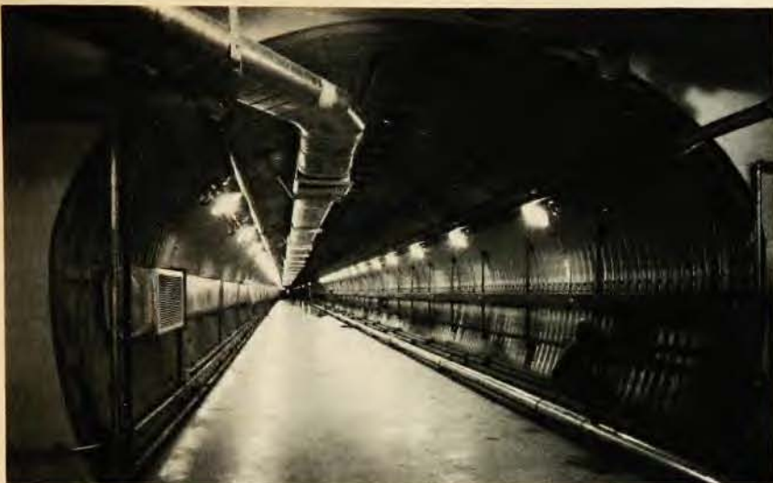
Underground tunnel near Livermore for the Advanced Technology Accelerator and adjoining experimental tank is 200 meters long. When completed this Fall, the 190 ferromagnetically loaded modules of this induction linac should produce repeated 10-kiloamp pulses of 50-MeV electrons, primarily for the study of charged-particle-beam propagation in air. The Experimental Test Accelerator, the 3-year-old, 2.5-MeV prototype for the ATA, is seen at right.
