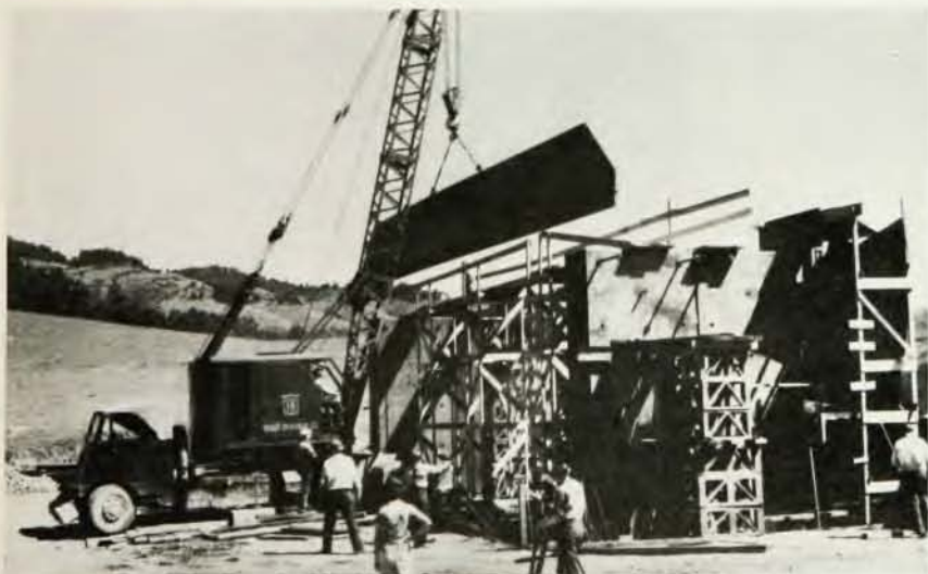
Construction of a building for the 184-inch cyclotron in 1941, on the Berkeley campus of the University of California. The building is still a part of the Lawrence Berkeley Laboratory.
