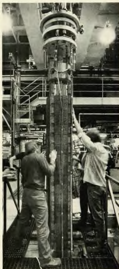
15-foot Palmer magnet for Isabelle undergoes a check at Brookhaven before it is returned to a Dewar for cooling to 3.8 K.
