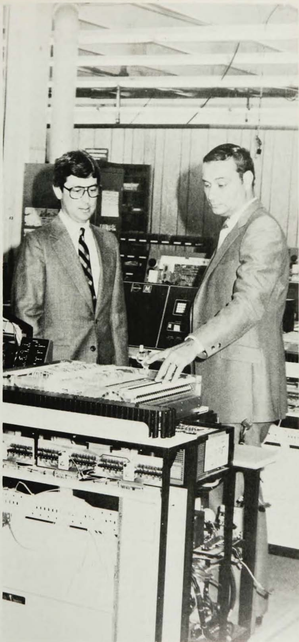
Clinical analyzer , capable of performing over two dozen chemical tests on blood serum, can process 120 samples per minute. Michael Molnar (right), who directs instrument research and development, is shown here with John Dorson, marketing manager for the analyzer.
