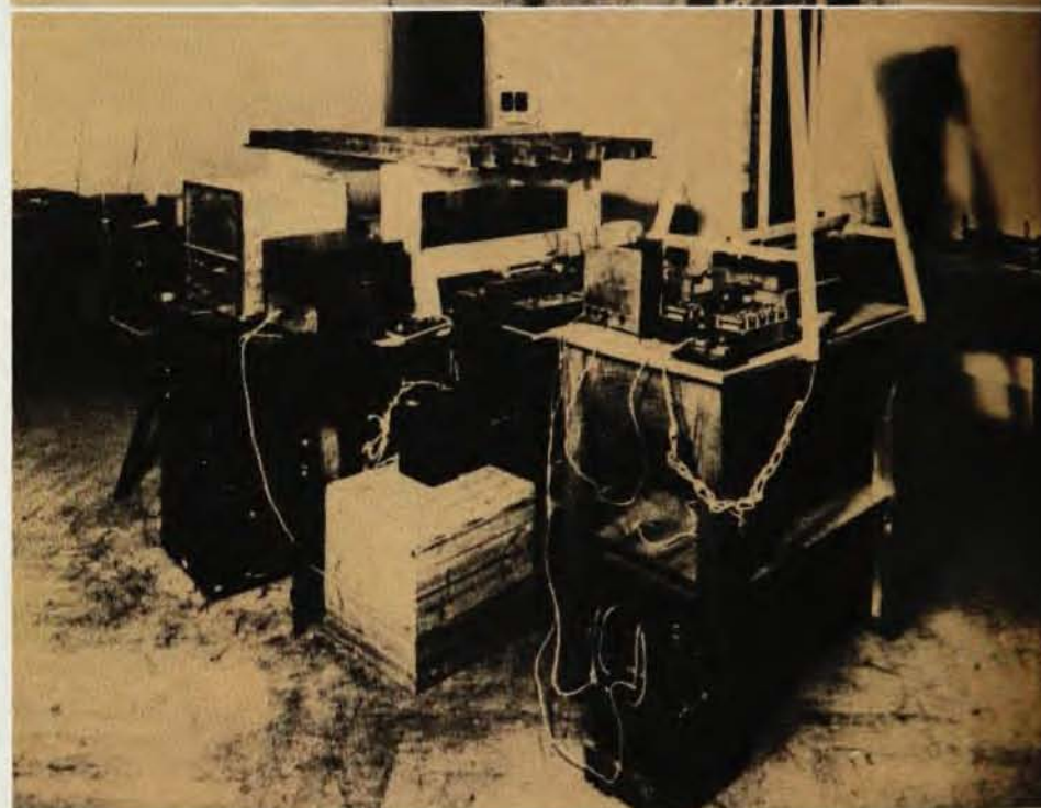
Experiment by author was first to use threefold coincidence and showed that cosmic ray particles could penetrate meter of lead. Figure 3.
