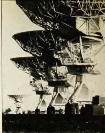
Very Large Array radio telescope. All 28 dishes have been built and are now being installed in a Y-shaped arrangement at the site near Socorro, New Mexico. When completed (probably by the end of the year), the VLA will have a maximum resolution, depending on its operating frequency, of 0.1–0.5 arc-sec. NSF expects to provide $5.2 million in FY 1981 for the operation of the Very Large Array.
