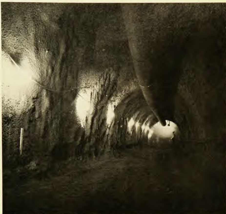
Construction of the ring tunnel at PEP , an 18 GeV \times 18 GeV electron-positron storage ring. Because of the variation in height of the terrain, parts of the ring enclosure are tunneled, parts are poured-in-place concrete. The interior of the tunnel walls is "shotcrete" and will be only slightly more regular in surface than they appear in this photograph. The ring has a 710-m. diameter.
