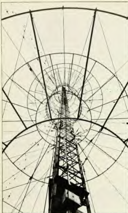
Antenna systems receive thorough treatment in J. D. Jackson's text; this monopole radio antenna developed by ITT Electro-Physics Laboratories applies the principles of electromagnetic-wave propagation discussed by the author.
