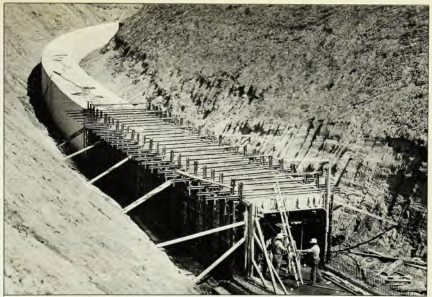
Tunnel construction is nearly completed at the PETRA electron-positron ring in Hamburg (see "Search and Discovery," PHYSICS TODAY, June 1976, page 17 for details). What new particle data will PETRA, PEP (being built at the Stanford Linear Accelerator Center) and other new accelerators produce? How will these data fit in with the gauge theories? (Photo courtesy of G.-A. Voss, DESY) Figure 1
