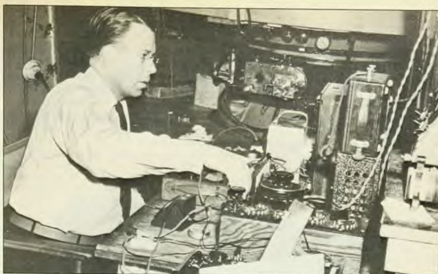
Ernest O. Lawrence sits at the controls of the mass spectrometer , which was constructed out of the 37-inch cyclotron in 1941. Without a jacket, this would appear an "at-work" shot, yet, according to Luis Alvarez, "we spent most of our time looking like garage mechanics." Figure 4
