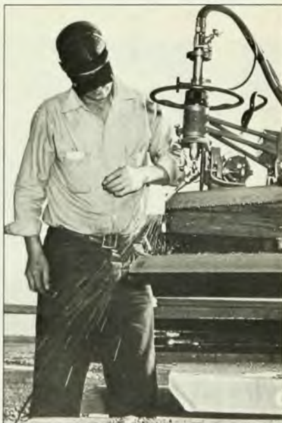
Another rare shot of a physicist at work is this graduate student at the University of California, Berkeley in 1940, who is torch-cutting bevels on a portion of the 184-inch cyclotron magnetic structure. The subject is Robert Wilson, now the director of Fermilab. Figure 5
