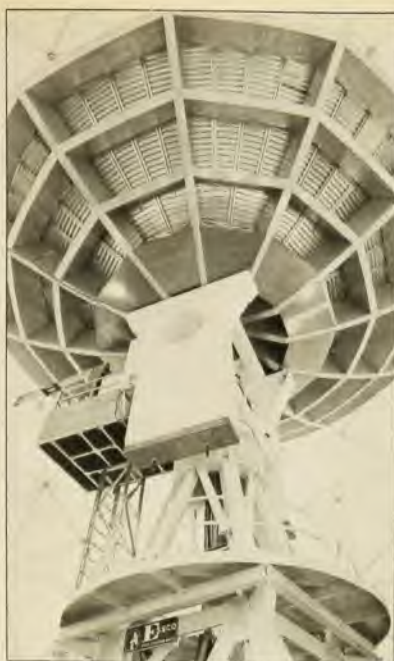
Millimeter-wave radio telescope at Five College Observatory. Photograph shows the box-beam back structure, pick-up arms and pedestal.
