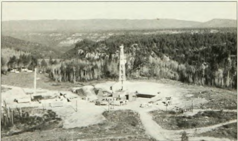
Site of geothermal experiments near Valles Caldera, N.M. Small drill rig is over the first hole (about 3 km deep); the larger one is in process of drilling the second borehole.
