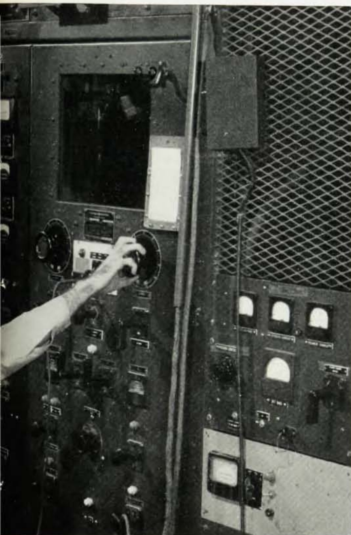
Final purification of radioactive iodine-131 is accomplished in this hot cell operated by remote control.
