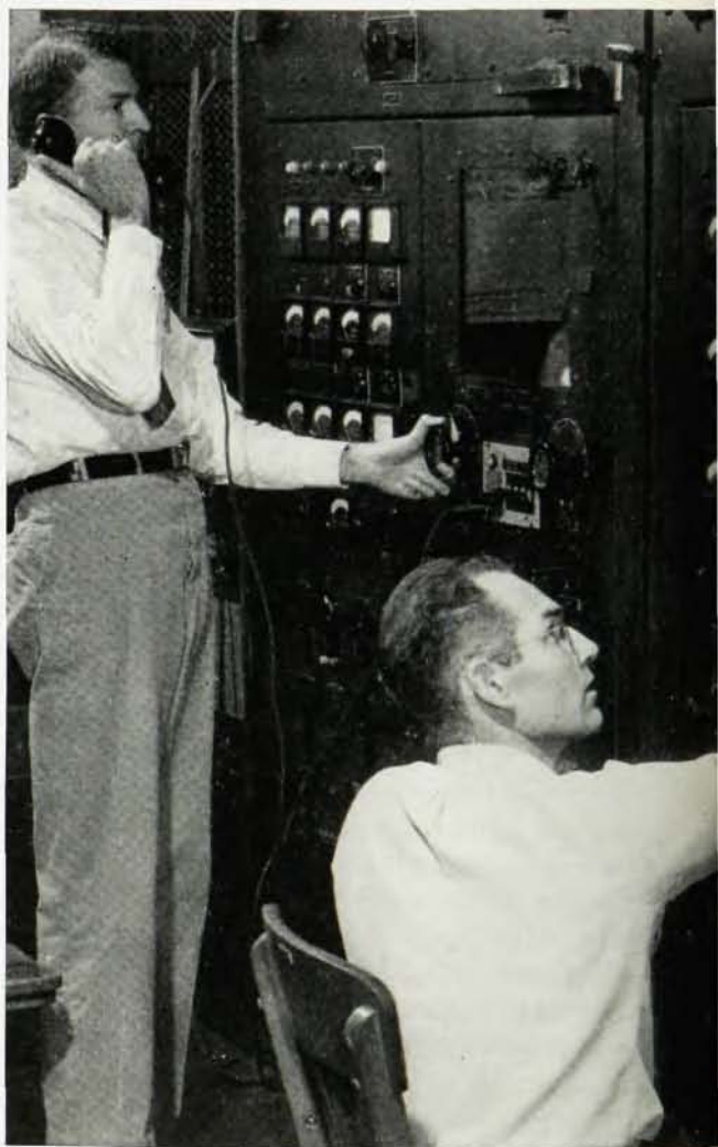
At the controls of the mass spectrographs (calutrons) engaged in enrichment of stable isotopes.
