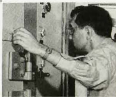
Final purification of radioactive iodine-131 is accomplished in this hot cell operated by remote control.
