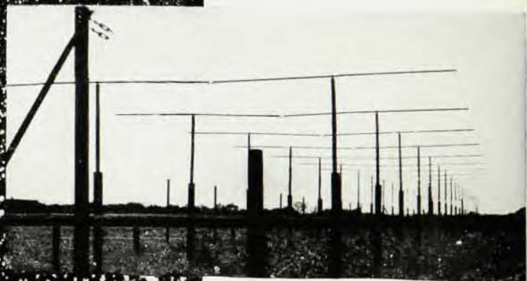
Western half of interference aerial system at Cavendish for locating galactic sources. Photo at the left is the Dark "S" nebula. Mt. Wilson Observatory photo courtesy of Hayden Planetarium.
