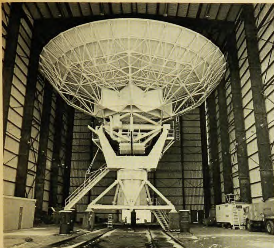
Second antenna in the Very Large Array is outfitted with electronics. By 1981 there will be 27 such 200-ton antennas, 82 feet in diameter, arranged in a Y shape with 13-mile branches.
