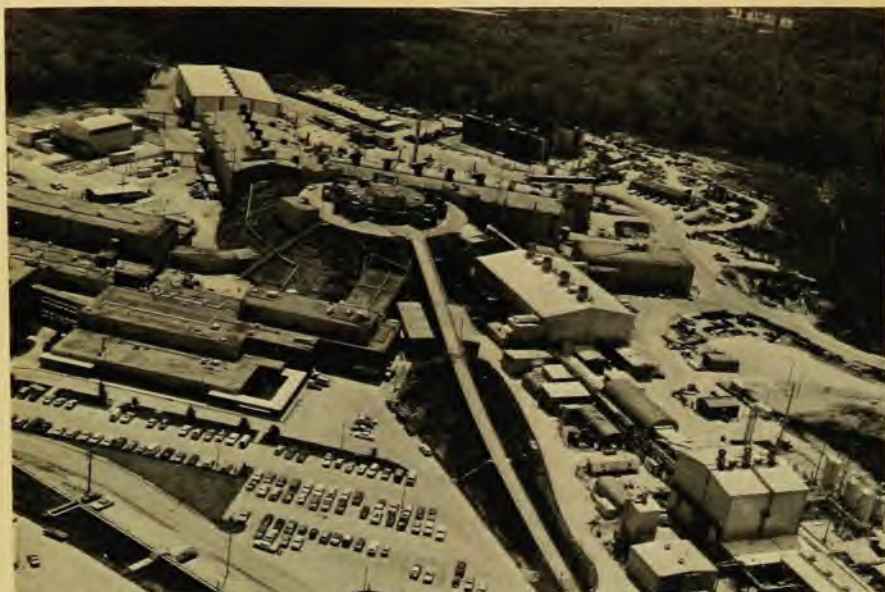
Argonne's ZGS complex includes neutrino beam line and 12-foot bubble chamber at lower right. Two halls for polarized-proton-beam experiments are at upper left.
