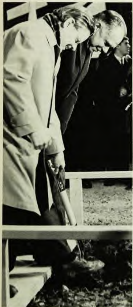
Groundbreaking in 1969 for the National Accelerator Laboratory at Batavia, Illinois, featured Robert R. Wilson, director, and AEC chairman Glenn Seaborg sharing shovel.
