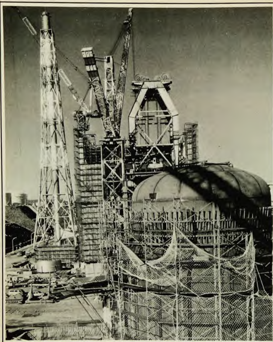
Nuclear reactor at Fukushima, Japan, under construction. One of six reactors on the site, this boiling-water reactor is a GE design in the 1000-MW range. US-designed reactors are sold in Japan, Spain, Italy and many other countries; at the same time the US is confronted with competition on world markets from French, Swedish, Japanese and Russian manufacturers.
