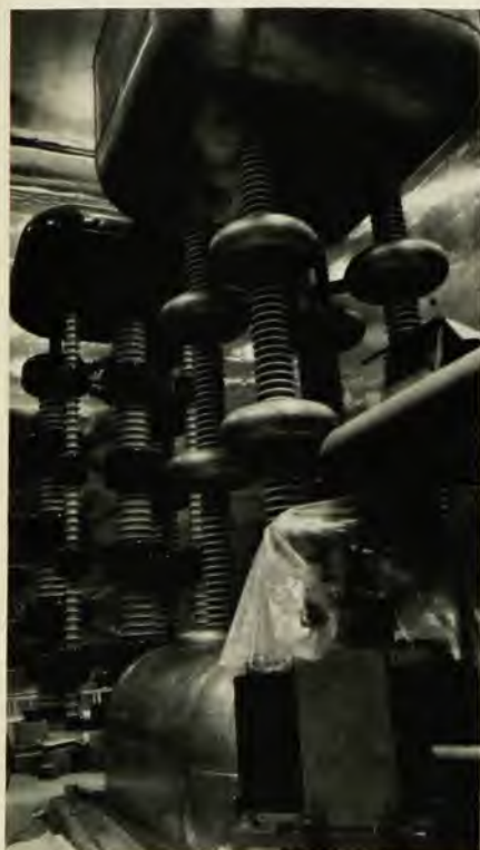
The ion production source for the Tsukuba synchrotron will be this 750-kV Cockcroft-Walton preinjector, moved from the University of Tokyo in 1971. Figure 4
