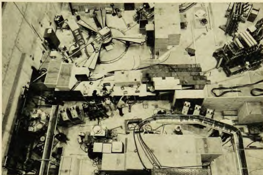
Proton hall at TRIUMF will have two beam lines (entering from lower left). This is part of a Canadian meson factory in Vancouver run by a four-university consortium. The other experimental area is a meson hall with two meson-producing targets and four experimental channels.
