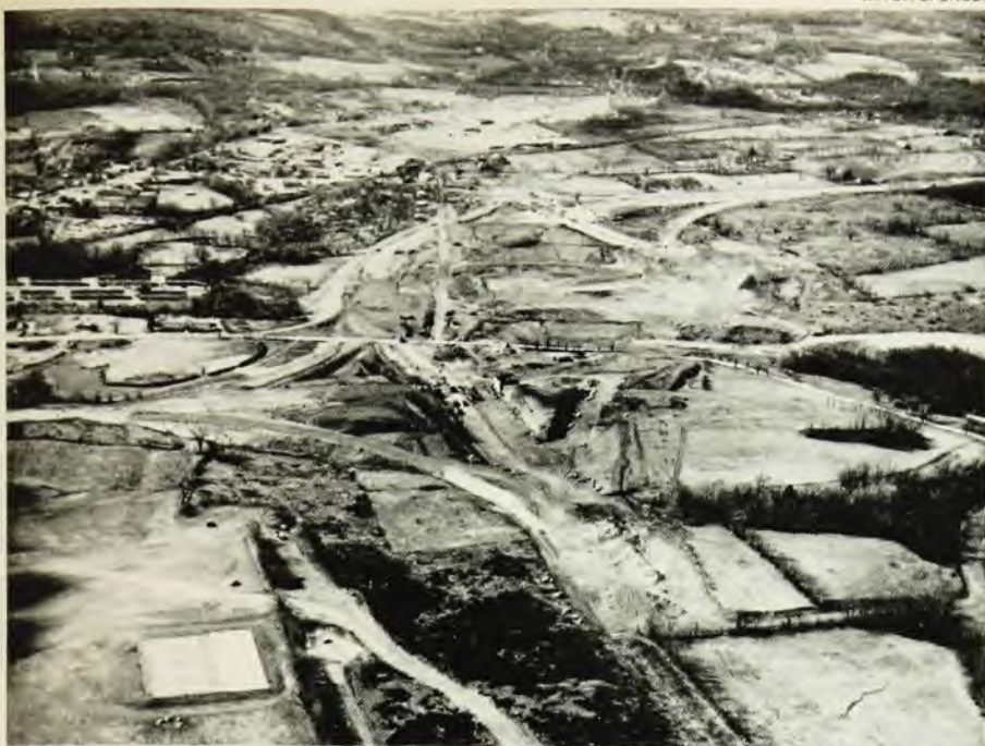
This mass of scarred earth marks the construction of a cloverleaf interchange in Bennington, Vermont, part of a new four-lane highway to replace an existing two-lane route. Robert Morris, a traffic engineer and transportation planner, worked with various public-interest groups to convince the 2nd US District Court that there is no need for the enlarged route, and the Court issued an injunction halting construction.
