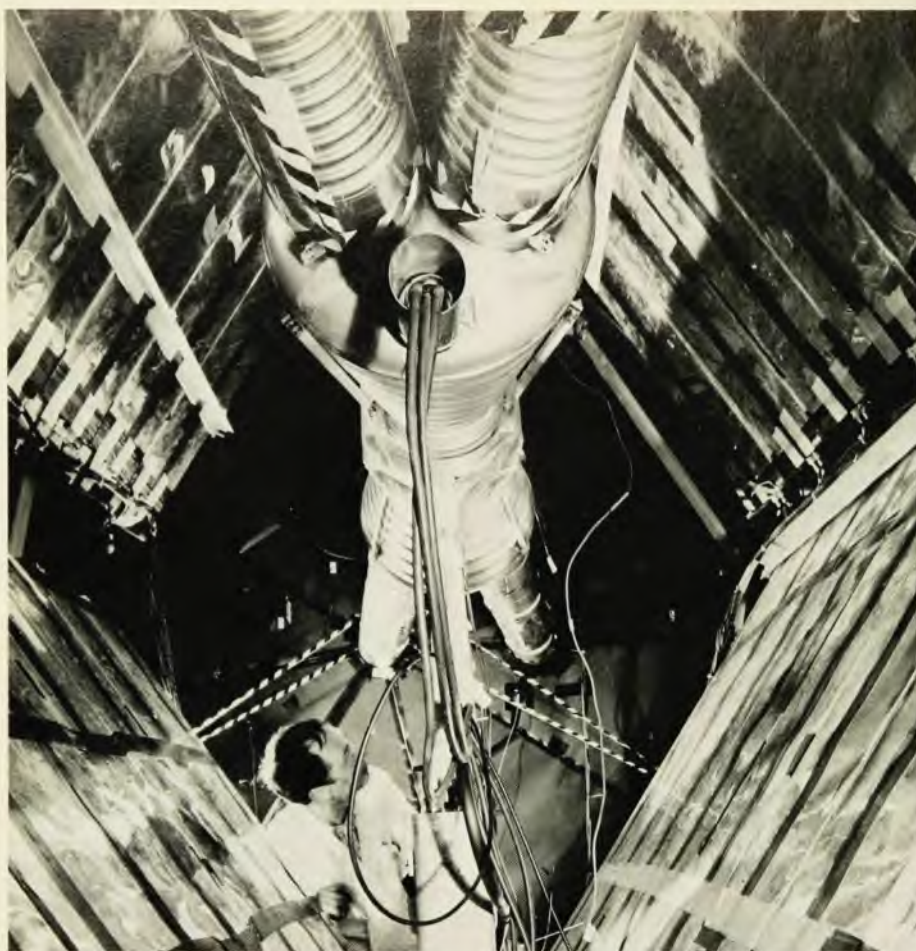
One of the intersection regions of the Intersecting Storage Rings at CERN, near Geneva, where the circulating beams of protons meet in almost head-on collision. Emitted secondary particles traverse the thin double stainless-steel walls of the vacuum vessel before entering the surrounding detectors. The discovery that cross sections rise with energy was made with the ISR.
