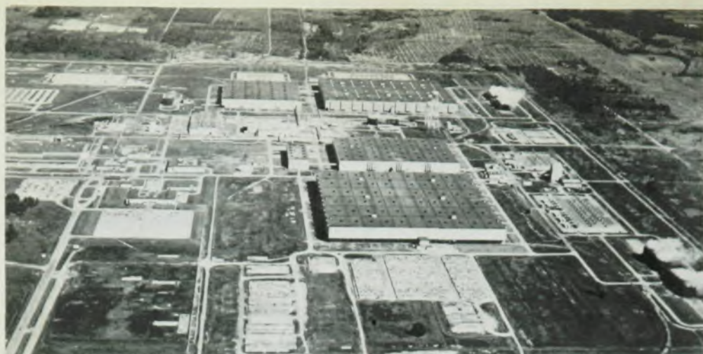
Paducah gaseous diffusion plant built and operated by the AEC since 1954 covers 74 acres and consumes 2550 Mw of power when functioning at full capacity. Figure 2
