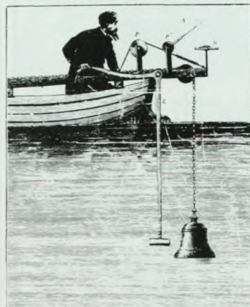
Underwater acoustics apparatus of the 19th century. This plate from Colladon's "Experiments on the Velocity of Sound in Water" appears in Lindsay's Acoustics: Historical and Philosophical Development .
