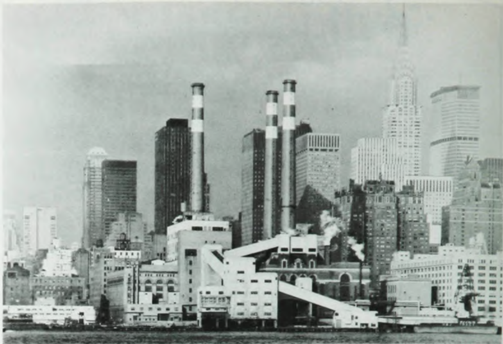
The Waterside Station in mid-Manhattan supplies 900 000 kW of electricity as well as 4.2 \times 10^6 lbs steam per hour to the Consolidated Electric Company's system. The plant's ten boilers burn natural gas and oil but not coal. (Photo: Edison Electric Institute)
