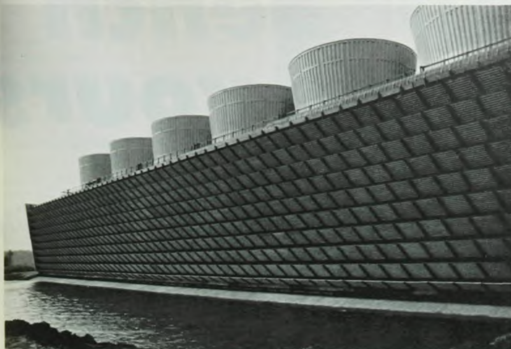
A new type of cooling tower that removes heat from water before it is returned to a lake. It is located at the Wilkes Power Plant near Jefferson, Texas. The plant produces 351 000 kW of power by burning natural gas. (Photo: Edison Electric Institute)
