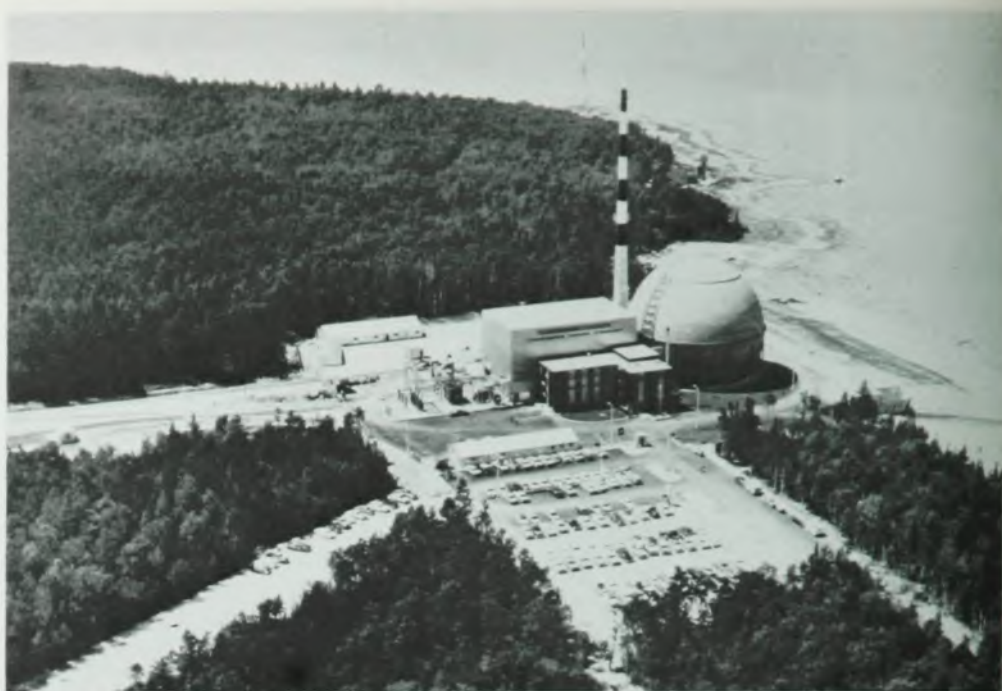
Big Rock Point Nuclear Power Plant is one of 15 boiling-water reactors currently in use. It has been producing 75 000 kW since December 1962 and recently set a record by giving 198 consecutive days of service. (Photo: Edison Electric Institute)
