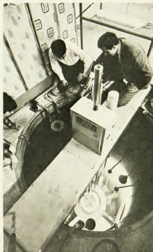
Mark II Triga reactor at Columbia University has been denied permission to operate. Core is viewed from top of installation through 16 feet of water. Grid plates that hold the fuel are seen at bottom.
