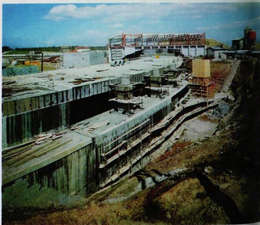
DETAIL OF RING CONSTRUCTION. Experimental Hall II is in background; it has flexible shielding arrangements that can be readily adapted to different requirements. Inside width of the ring tunnel is 15 meters; inside height is 6.5 meters. Some of the 1 million tons of rock and soil removed during the year-long excavation of the ring will cover it with about 4 meters of shielding.
