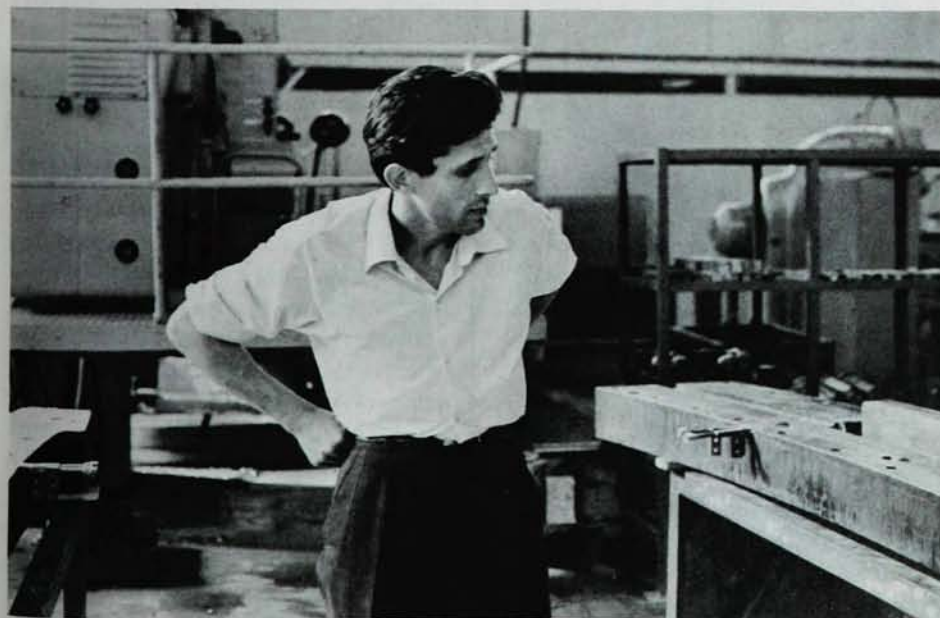
VADIM AUSLANDER WITH SOLID-STEEL MAGNETS, which are being built for air-core ironless synchrotron, part of the 25-GeV proton-antiproton storage ring.
