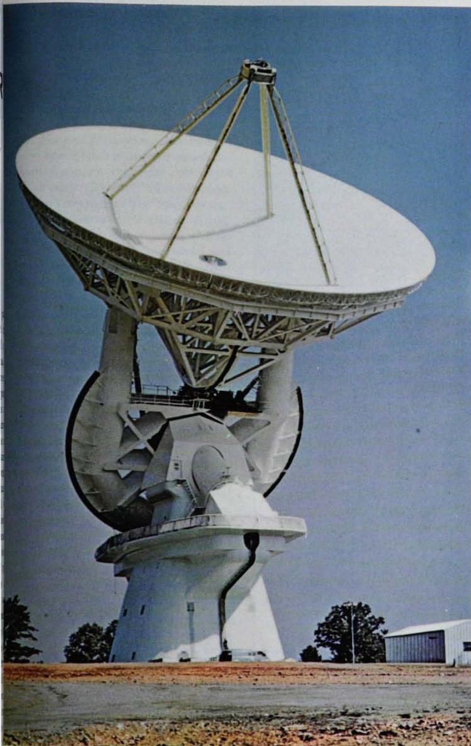
RADIO TELESCOPE at the National Radio Astronomy Observatory, Green Bank, W. Va. This 140-foot (43-meter) dish has been part of long-baseline systems that include radio telescopes in Massachusetts and Onsala, Sweden. —FIG. 1
