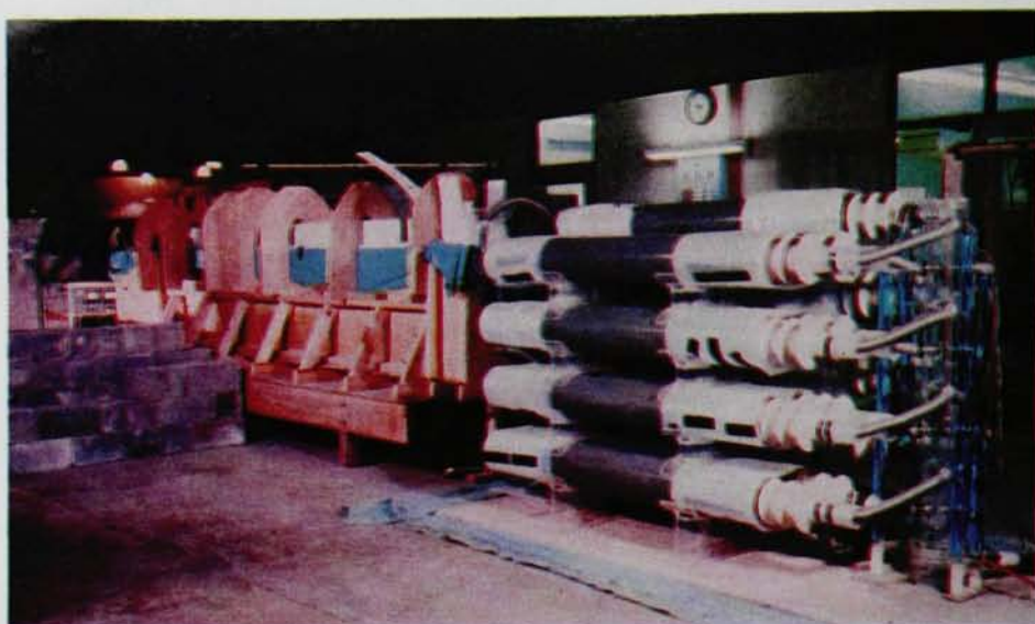
HIGH-INTENSITY ELECTRON ACCELERATOR at Cornell. Marx generator (right) erects a 700-kV pulse in about 300 nanosec. Then Blumlein transmission line (left) is charged to 500 kV in about 1 microsec and the energy is discharged.
