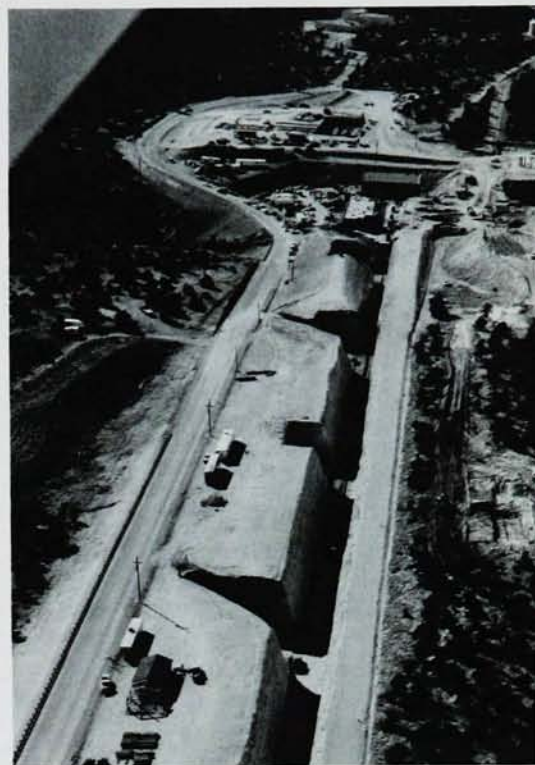
LOOKING WEST along beam-channel tunnel toward injector building. Equipment test laboratory is at top of picture; construction of a lab-office building has begun in the cleared area.
