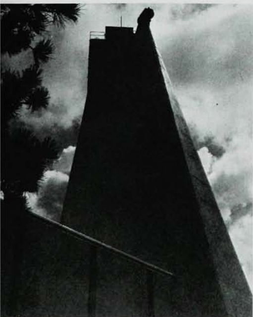
AIR FORCE SOLAR TELESCOPE is 111 meters high. The optical system is evacuated to 0.250 torr.
