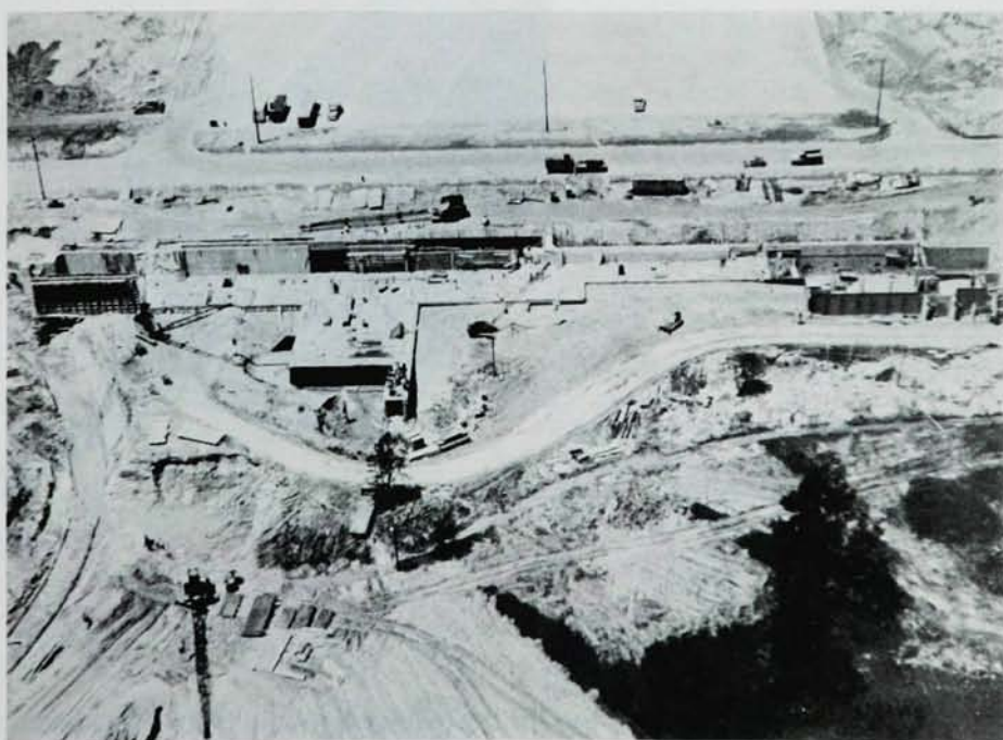
CONSTRUCTION PROGRESS AT BATAVIA. Building for the linear accelerator, which accelerates protons from 750 keV to 200 MeV, is at rear. At left is the enclosure for the booster synchrotron, which accelerates the 200-MeV protons to 10 GeV. Weisskopf panel says completion of 200-GeV accelerator should have highest priority for near future. Machine is scheduled for operations in mid-1972.
